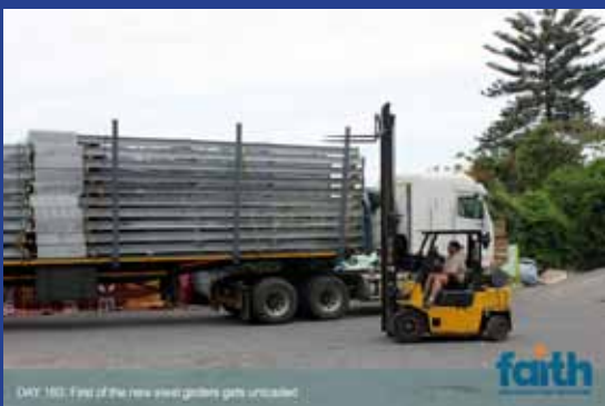
DAY 183: First of the new steel girders gets uncrated.
